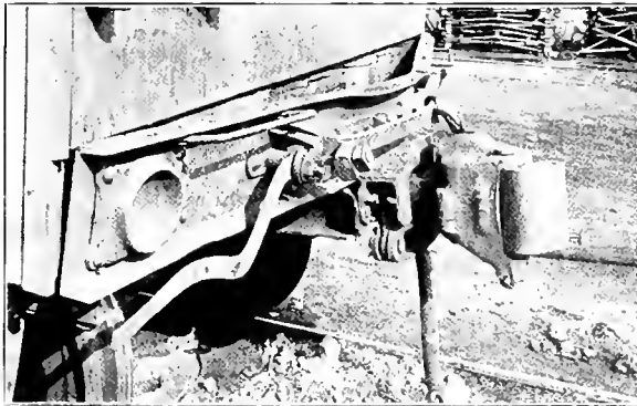
Fig. 1—Weak Draft Sill Pulled Out
